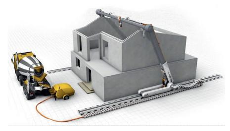
**Figure 3.29.** Artist impression of the so called 'Contour Crafting' technology that enables Digital Fabrication of buildings. (Grozdanic 2014)
